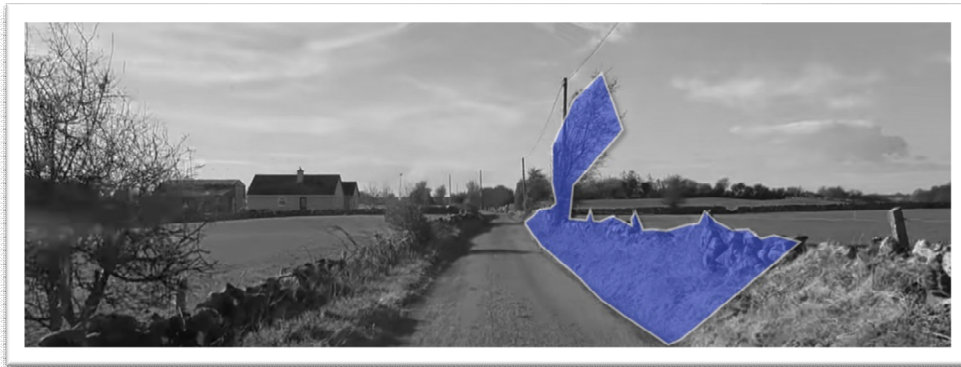
Figure 2.3 – Foliage in Ditch Obscuring Sightlines to Right for Emerging Vehicles
